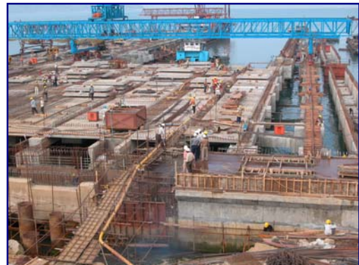
Project Seabird; Pier No. 1 & Shiplift Piers CALTITE pre-cast & in-situ marine concrete
