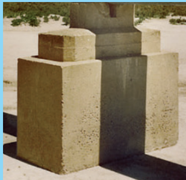
Cast in 1962 to replace damaged chair, with Caltite - condition after 40 years
