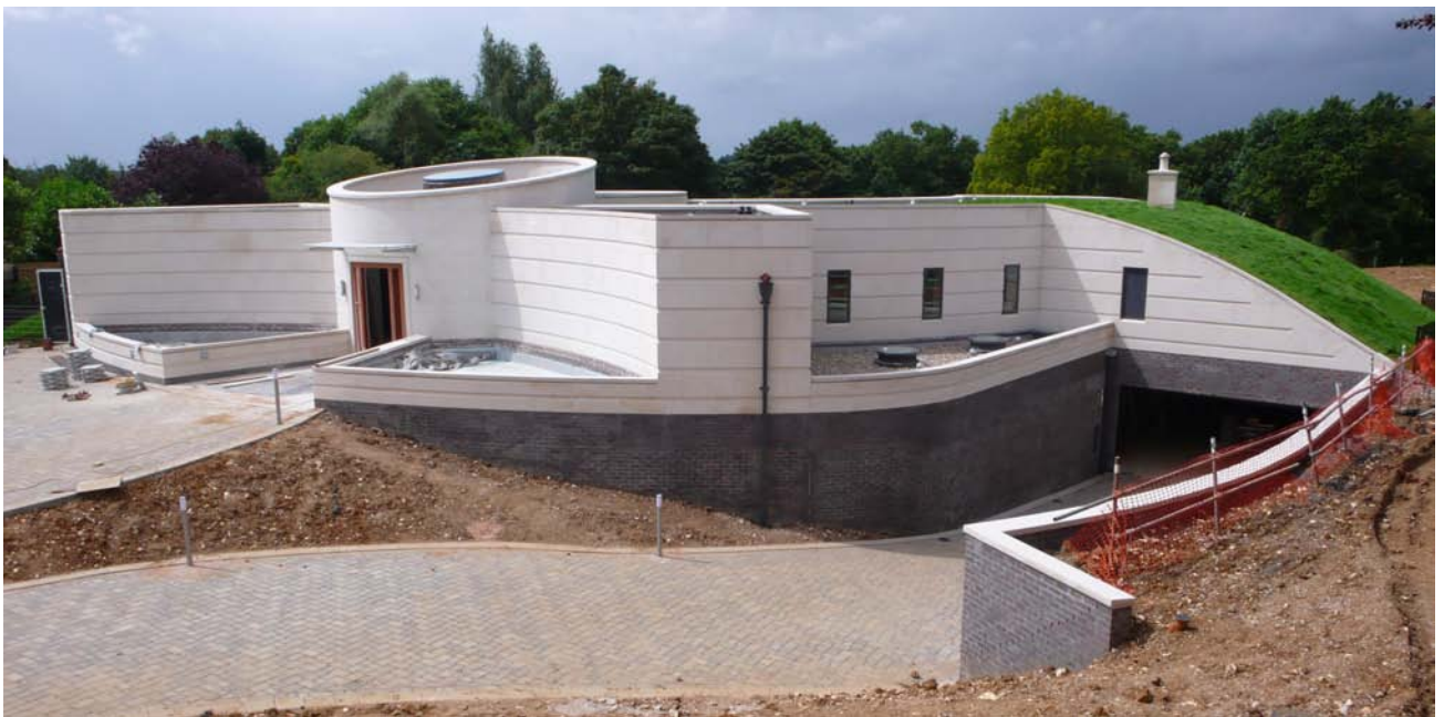
Caltite basement garage under green roof
