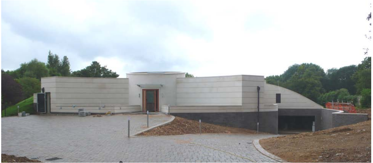
Swimming pool is under sloping green roof to the left
