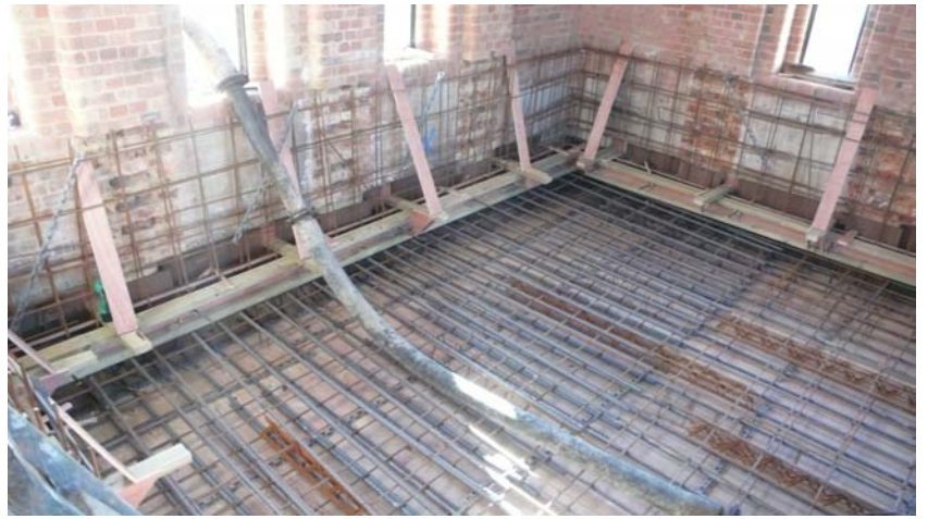
Suspended Swimming Pool on 4 th floor, 75ft up!
