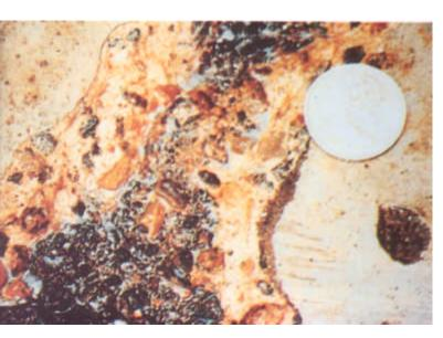
With constant traffic over the slab, the epoxy coating was not able to bridge micro-cracks which appeared early in the unreinforced screed. (Today's Everdure Caltite acid-proof floors/screeds may include specialised crack-control fibres). These photos show the effect of 20 years acid etching on the "faces" of these cracks, only mildly exacerbated by abrasion / impact from wheeled & forklift traffic.
