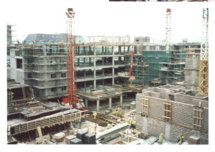
**CENTURY HOUSE, ST HELIER, JERSEY**1,893m³ of Caltite System concrete used to waterproof the basement slab and retaining walls
